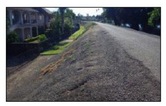
Erosion of Levee Slopes:
